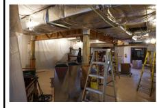
New ceiling tiles will be installed after the HVAC, electrical and other wiring is completed.
